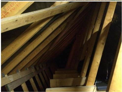
Plate 22 - BG4 -Building 1 -Interior view of roof showing modern trussed roof.
